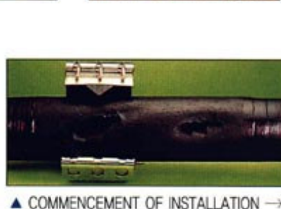
▲ EMERGENCY REPAIR SITE FOR UNDERGROUND WATER SUPPLY LINE
