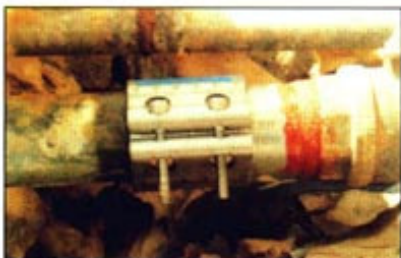
▲ COMPLETION OF CONNECTION WITH STEEL PIPE & DUCTILE PIPE
