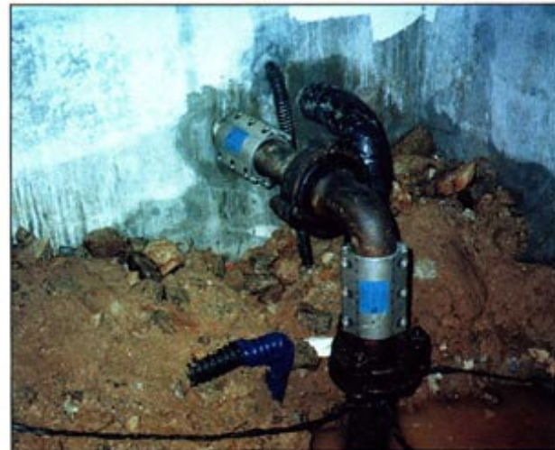
▲ REPAIR OF A LEAKING WATER SUPPLY LINE IN AN APARTMENT BUILDING
