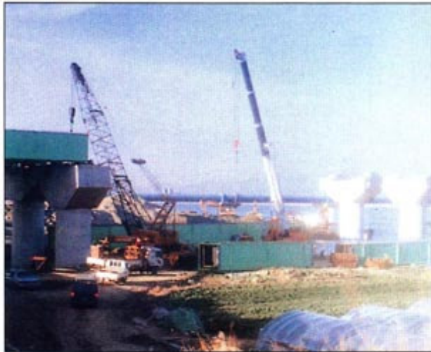
▲ LARGE WATER SUPPLYING PIPELINES
